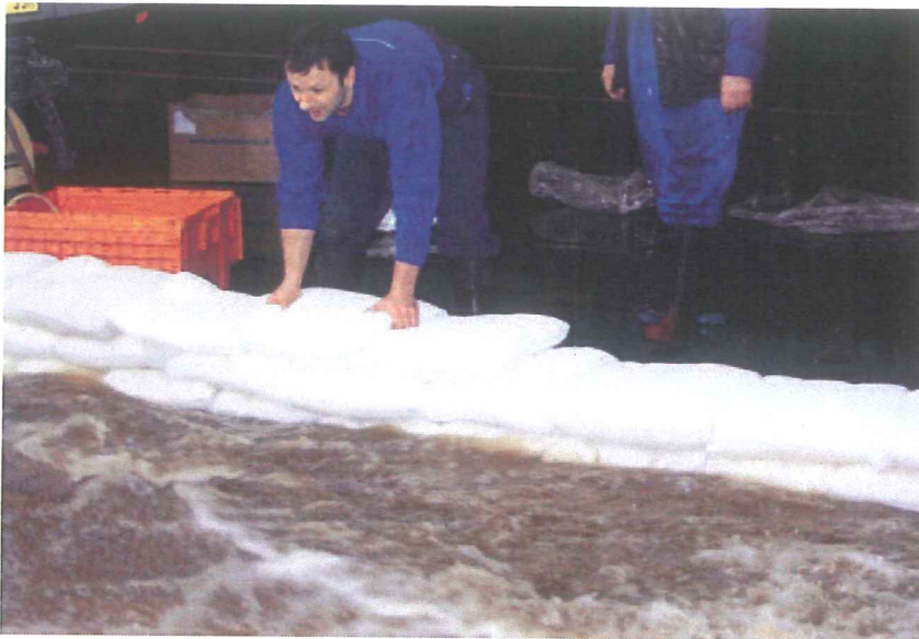
Dam clever: the Floodsax absorb water and then protect against flood
